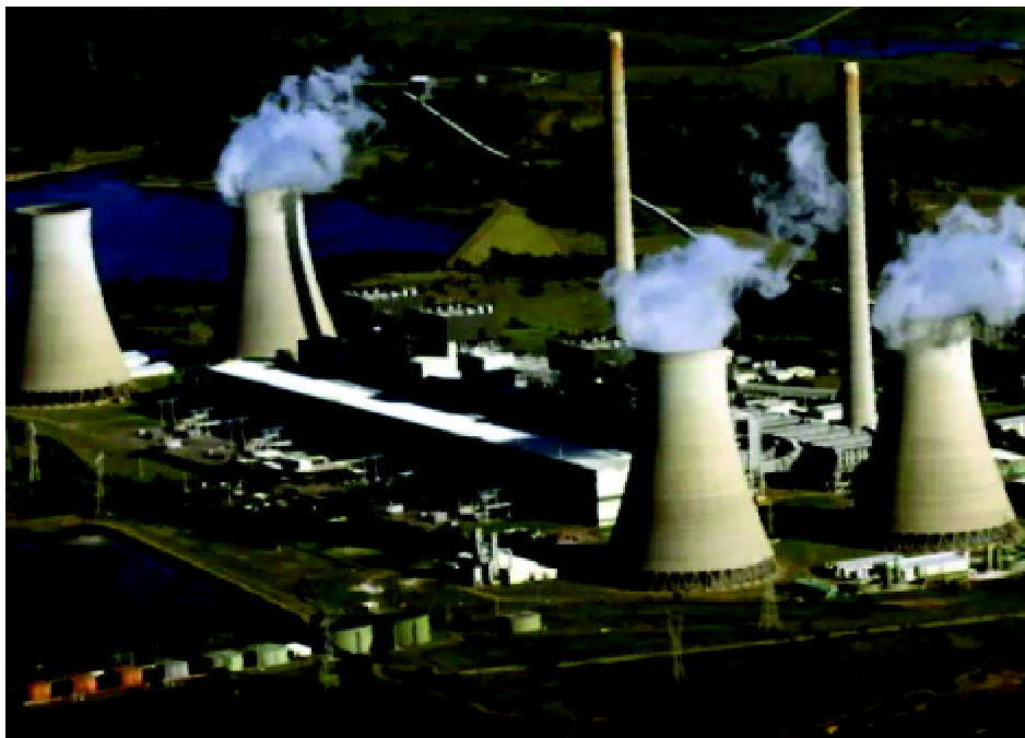
Newcastle power station.
